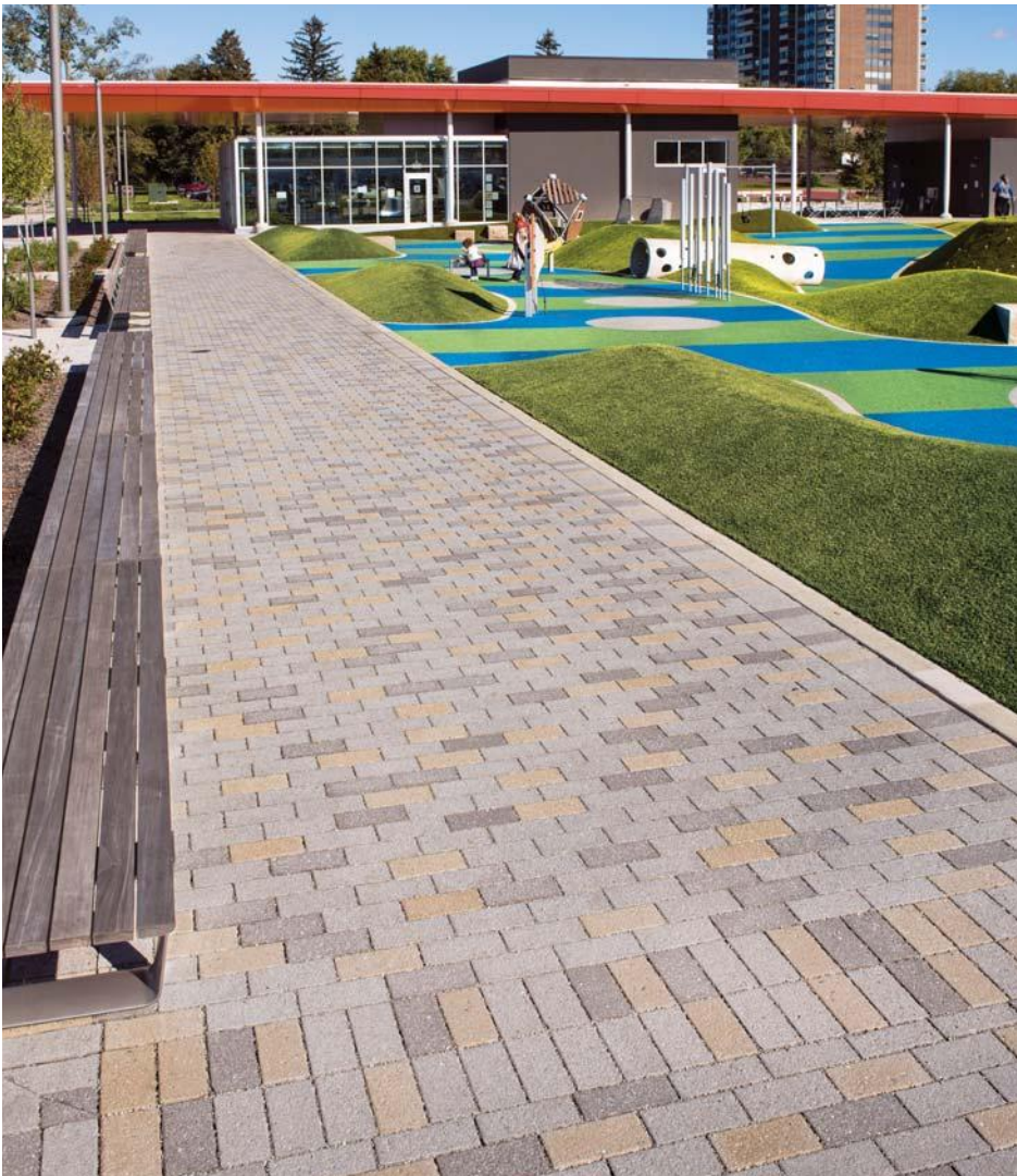
Tarkington Park, Indianapolis, IN; Owner: City of Indianapolis, IN; Architect: Rundell Ernstberger Associates; Size & Color: Permeable 4 1/2" x 9", Charcoal, Limestone Gray, Cream; Finish: Tudor®
